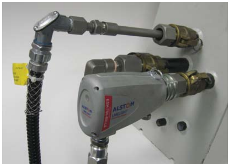
Flame Sensor Head of the LIMELIGHT Exacta Ignitor Scanner shown with oil side ignition system
